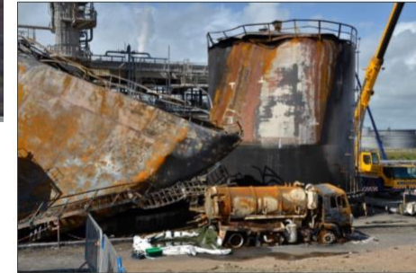
Figure 11 Post-incident – tank 17T302 minus vessel roof
